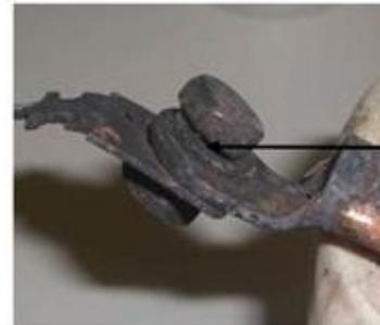
Washer located under bolt head. No spacer between lug and fuse blade
